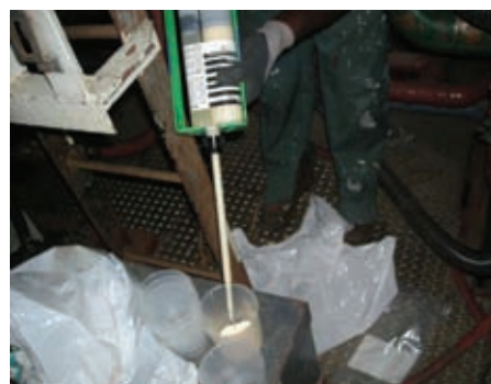
Fig. 5: Cartridges worked well for touchup, especially with several painters at once doing touchup work
