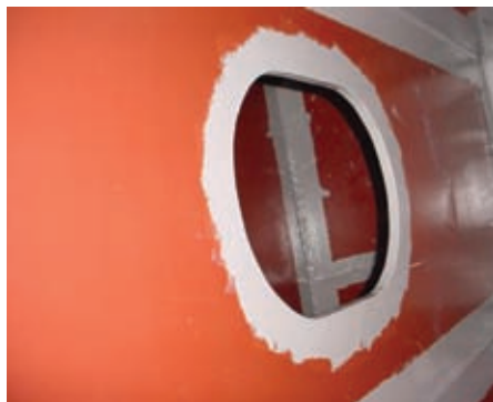
Stripe coat in ballast tank at newbuild stage Courtesy of Euronavy
