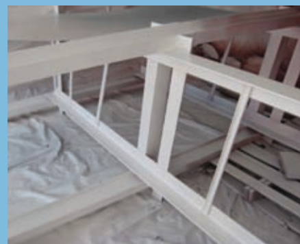
Fig. 1: Mockup for hands-on training of painters before starting the work Figs. 1-6 courtesy of NSRP “Fast Track” study
