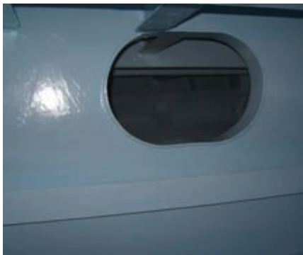
Fig. 7: DFTs on the first tanks were as high as 50 mils on the deck but for all other tanks, dfts were in the specified range of 20-30 mils in all locations.
