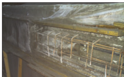
Fig. 4: Conventional concrete repairs and installation of remedial post tensioning tendons
