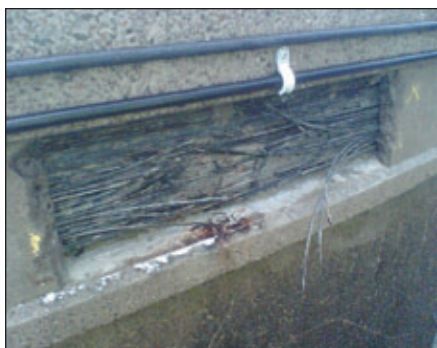
Fig. 3: Temporary tendons installed around the dome band
