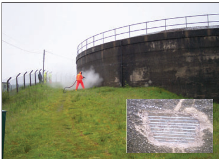
Fig. 1: Hydrodemolition to remove gunite overlay on tank walls. Inset: close-up of exposed wires.
