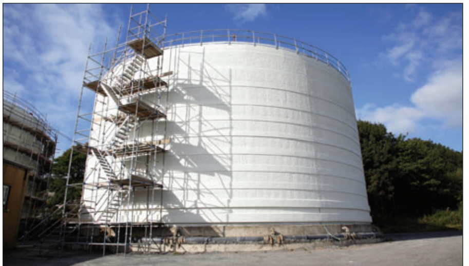
Top: Inspecting the tank Bottom: Final protective coating applied All photos courtesy of the author
