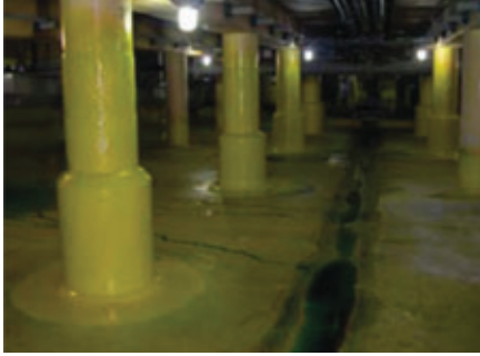
Fig. 6: Completed column repair
