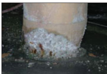
Fig. 1: Typical column degradation. Photos courtesy of the authors.
