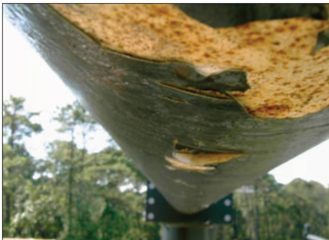
Fig 4: A close view of the surface beneath peeling paint on the underside of the mast arm in Fig. 2. The galvanizing is depleted and the steel substrate is corroding.
