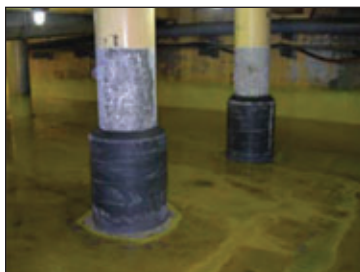
Fig. 5: Columns after removal of forms
