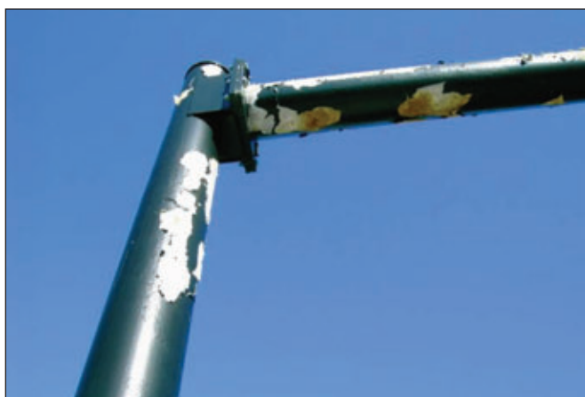
Fig 1: Coating peeling from the post and horizontal arm of a galvanized mast arm. The exposed surfaces contain white and red corrosion products.
