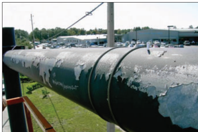
Fig 3: Appearance of failing coating on the side of a horizontal arm.
