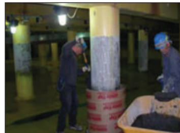
Fig. 4: Pouring of the polymer concrete
