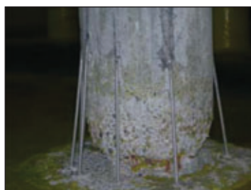
Fig. 2: Stainless steel rebar bent and grouted into the channels
