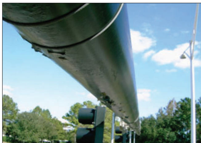
Fig 2: Peeling coating on the underside of the horizontal section of a galvanized mast arm.
