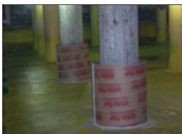
Fig. 3: The forms placed around the column
