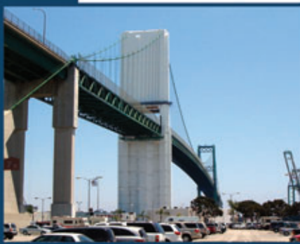
Vincent Thomas Bridge
