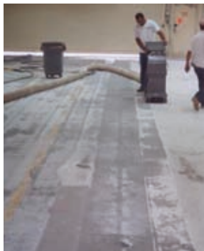
Surface Preparation (first of two passes)
