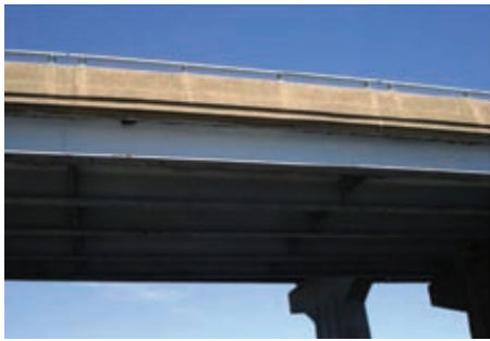
Photo 3: SP 2/Alkyd/epoxy/urethane coated span after 20 years.
