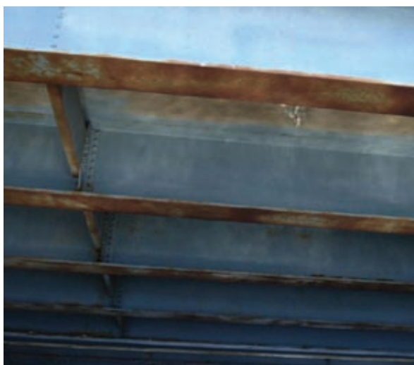
Photo 2: WBIOZ system with good condition of web, but poorer condition of bottom flanges
