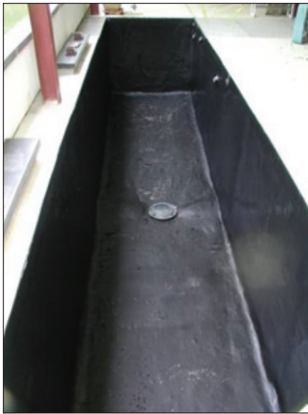
Fig. 2: A complete job. The floor is done after the walls are done.
