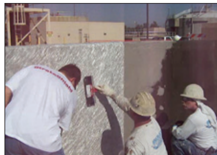
Fig. 2: Applicators smooth the fiberglass sheet into the wet basecoat.
