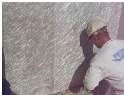
Fig. 3: Fiberglass sheet before the application of the saturant coat
