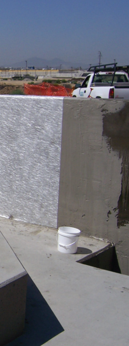
Interior wall of secondary containment shows the progression of the wet-on-wet lining process. From right to left: the dark area is primed, the light gray area is basecoated, the first panel of fiberglass is laid into the wet basecoat, and the last four panels are saturated.
