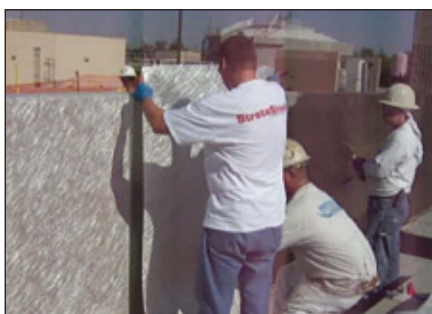
Fig. 1: Foreground: Fiberglass sheet is laid onto the wet basecoat (light gray area). Background: The basecoat has been applied over the wet primer (dark gray).
