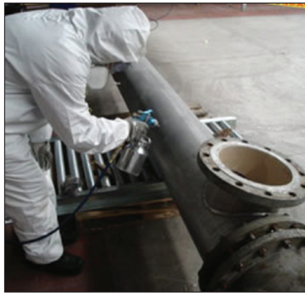
Some fall hazards can be eliminated by bringing the work down to the ground. Courtesy of the author
