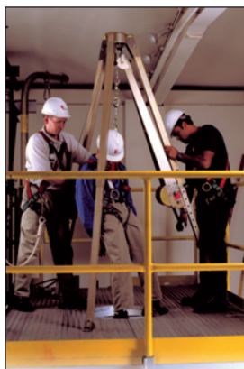
Confined space entry and retrieval system in use for training. Photos courtesy of MSA
