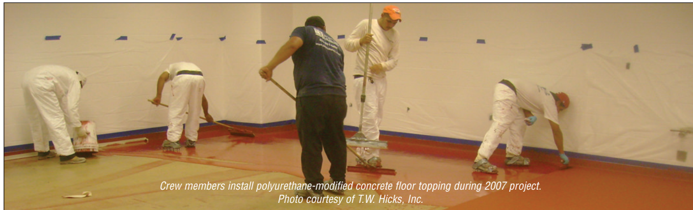
Production area of the newest facility, with floor topping installed in 2007 Photo courtesy of T.W. Hicks, Inc.
