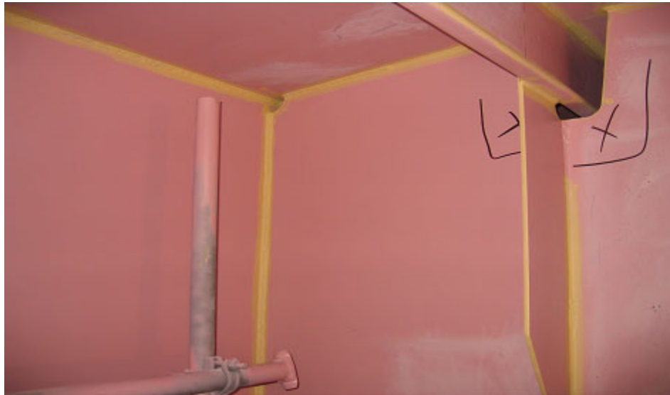
Photo 5 Typical example of good stripe coating. Note the care employed not to over build.
