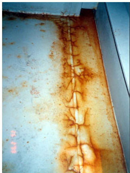
Photo 1 Typical example of cracking at weld
