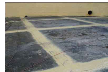
Fig. 3: Joint treatment in Tank 2 before final lining application
