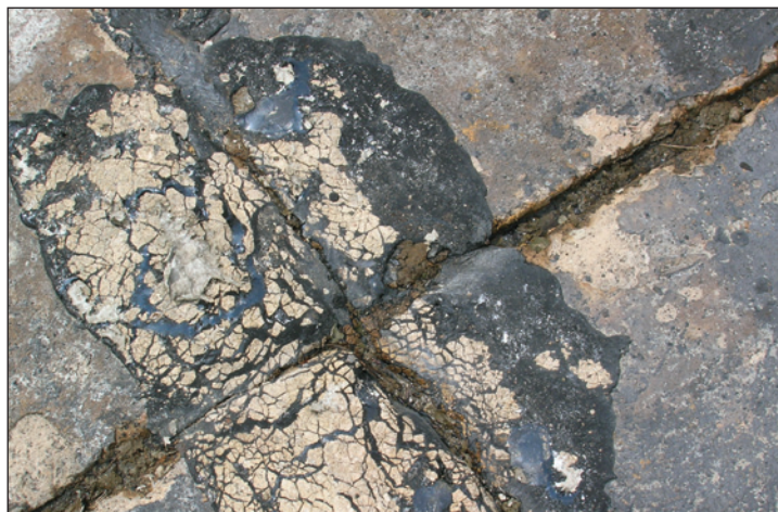
Fig. 2: Concrete control joint with caulking and asphalt-based patching material, later removed
