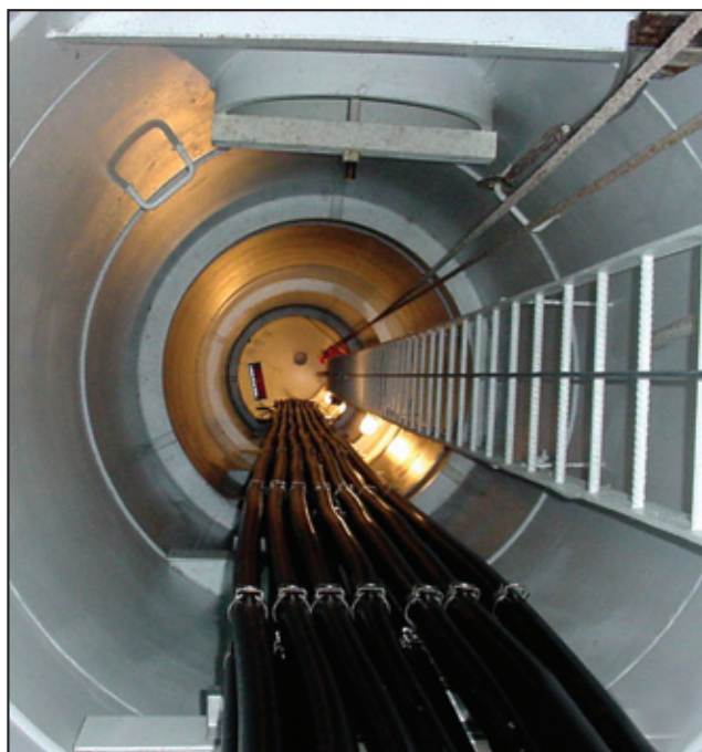
Fig. 2 (above): By keeping the coaxial cables together and aligned opposite the ladder in this tank tower, the cable installers preserved access to the tank for maintenance or other needs.
