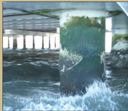
Fig. 8: Bent 694, polyurea delaminating from the pile
