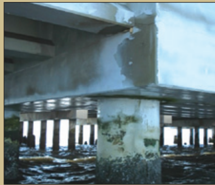
Fig. 5: Delaminated polyurea on corner of pile cap
