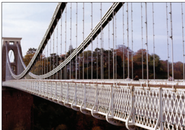
The Clifton Suspension Bridge, completed in England in 1864, originally used cast iron suspension chain, which was replaced with steel cable.
