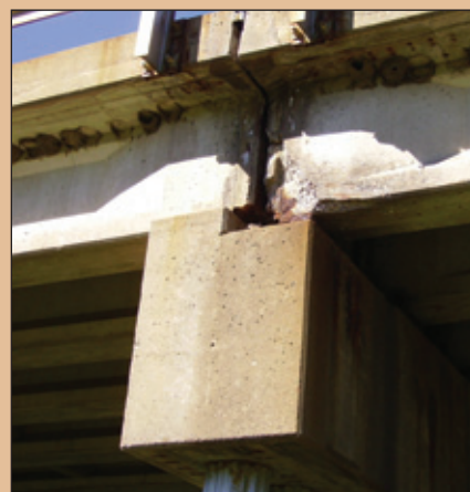
Interior and exterior views of corroded, contaminated girders
