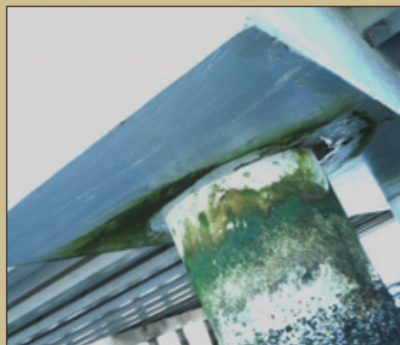
Fig. 1: Pile cap/pile interface, with polyurea delaminated from the joint. Photos courtesy of the authors
