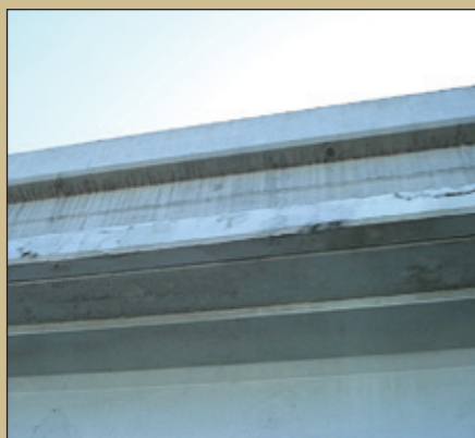
Fig. 3: Edge of the deck and barrier rail on top of a girder
