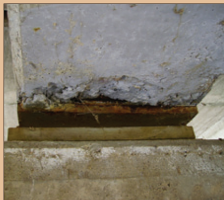
Corrosion at concrete beam end with salt infiltration Photos courtesy of the authors
