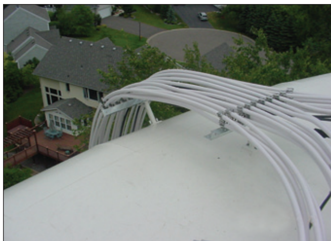
Fig. 5: On the roof of a ground storage tank, this manufactured, colored coaxial cable installed over a shop-painted mount (on the left) will have a longer service life than a painted cable. Note that the studs holding the bracket have white plastic caps that prevent rusting. Holding the cable on top of the mount is a galvanized z-bracket.
