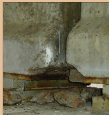
Degradation at beam ends
