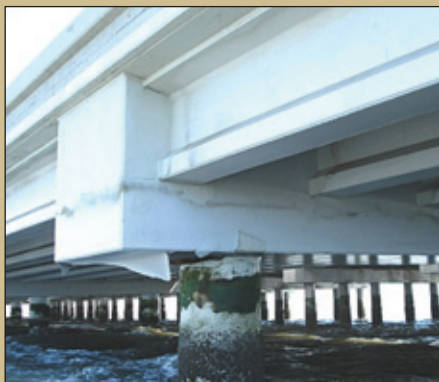
Fig. 7: Polyurea delaminated with no primer evident on the pile cap.
