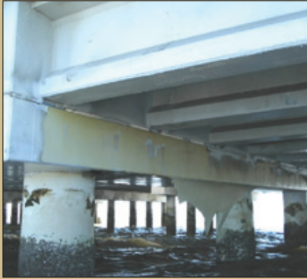
Fig. 4: Pile cap looking from the north. Notice the yellowed polyurea.
