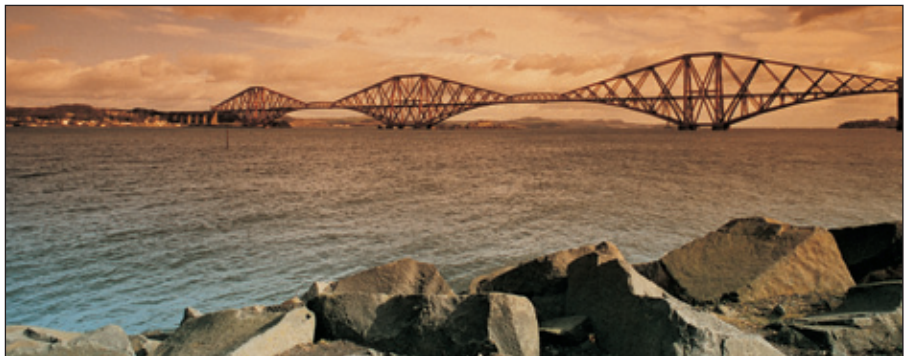
The Forth Rail Bridge in Scotland, a steel cantilever bridge completed in 1890. Courtesy of Peter Morgan
