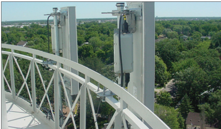
Fig. 4: This galvanized antenna attachment on a water tank handrail eliminates damage to the paint and requires minimal maintenance.
