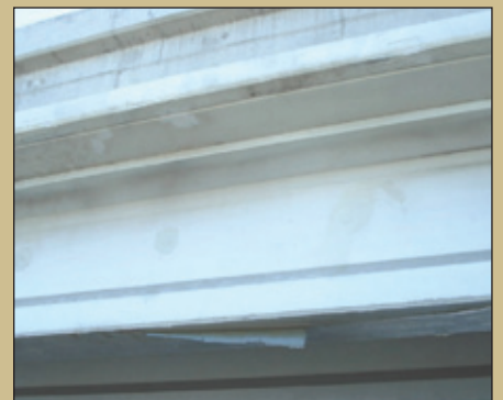
Fig. 6: Polyurea peeling away, no indication the primer was present
