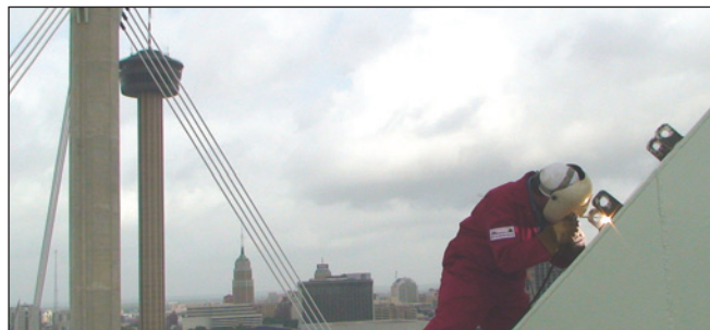
Welding the rope anchor points, or “pad eyes”, to the Alamodome roof. Photo by Howard Wall, courtesy of MHT Access Services Inc.
