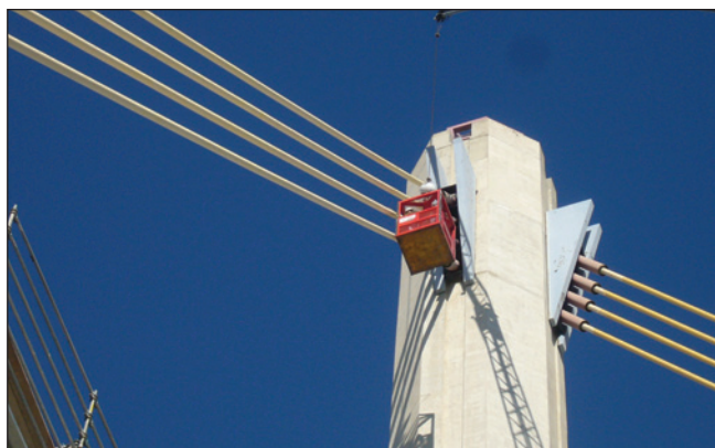
Two-man basket, suspended from crane, used to access upper cable runs from the mast column to the corners. Courtesy of Paradise Painting, Inc.
