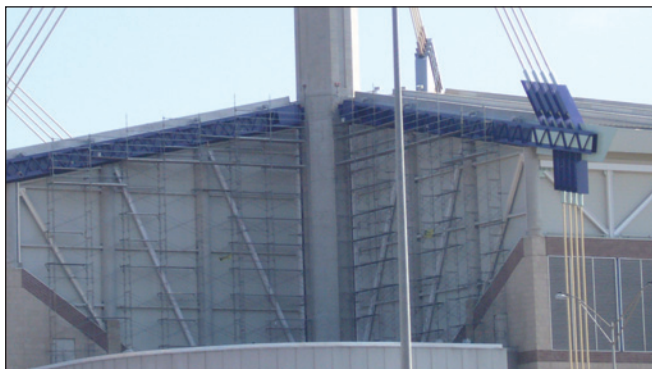
Scaffolding erected to access eyebrow trusses. To the right is an outer cable. Courtesy of Paradise Painting, Inc.
