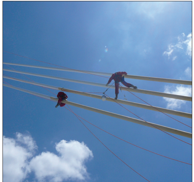
Rope access workers paint cable sheaths. Photo by Jesse Cantu III, courtesy of MHT Access Services Inc.
