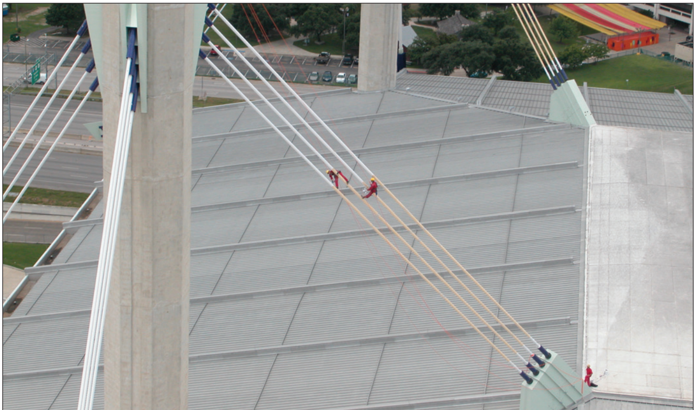
Rope access workers painting the “inner” cables at the Alamodome. The cables connect the roof to exterior 300-foot mast columns. Note the tie offs below, above, and on the workers. Photo by Howard Wall, Courtesy of MHT Access Services Inc.
