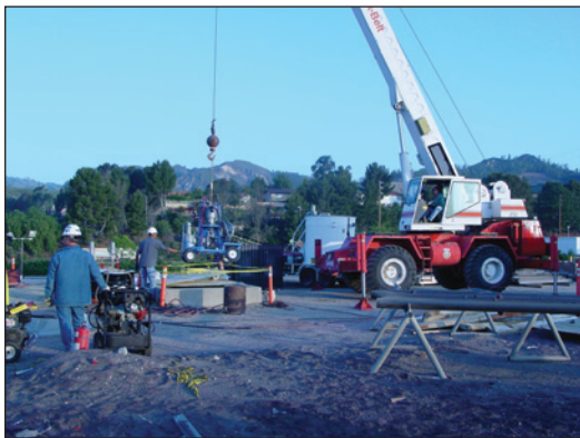
Plural-component spray system being lowered into shaft leading to water transmission tunnel. Safe practice is needed even before work begins.
