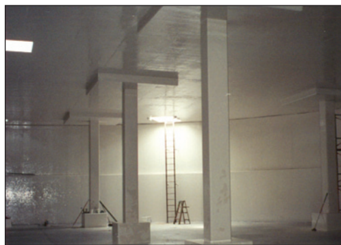
Potable water tanks like this one can be confined spaces and require special procedures, even with plural-component spray-applied epoxy. All photos courtesy of RLS
