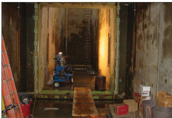
Plural-component spray equipment inside water treatment structure prior to spray application.
