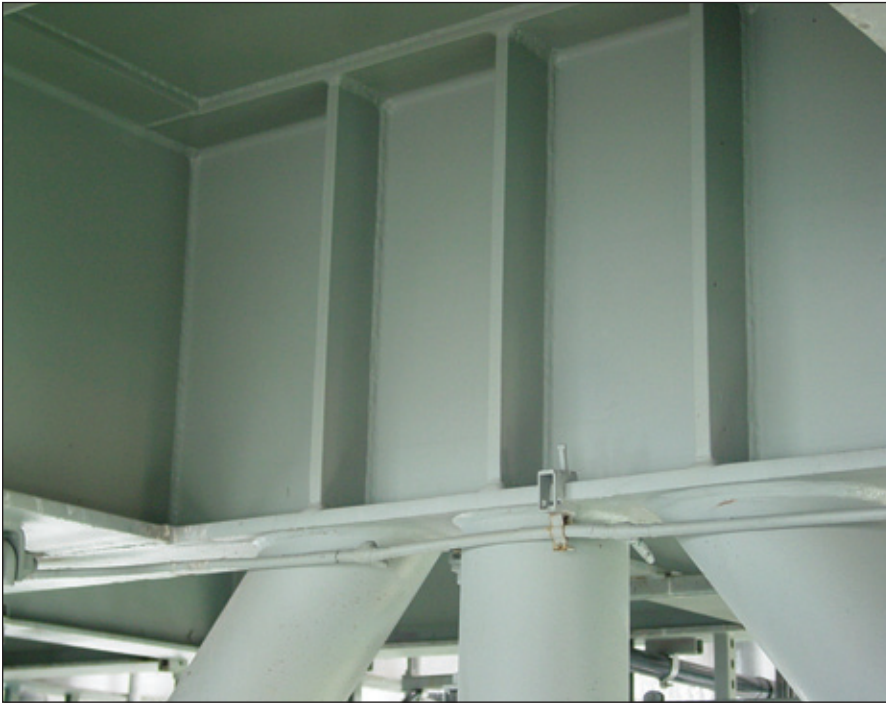
Structural steel beneath main loading platform showing no chalking or edge failure
