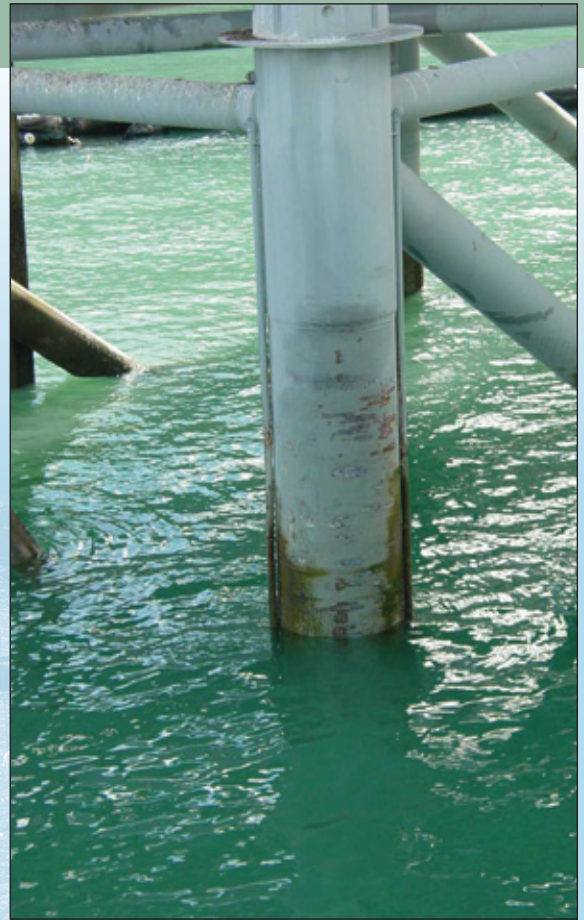
BOC piling in splash zone showing mechanical damage and marine growth
