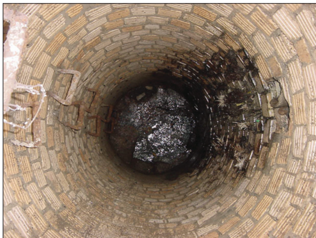
Confined space procedures must be followed to rehabilitate this sanitary sewer manhole.
