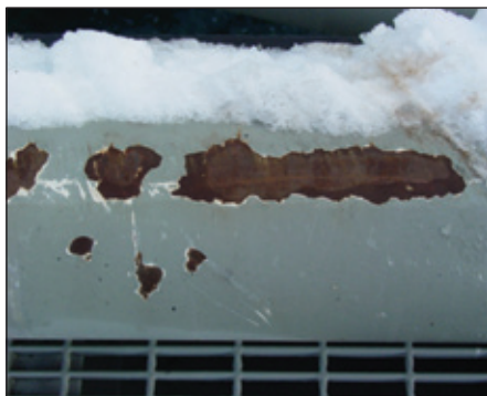
Coating failure on berthing dolphin bull
