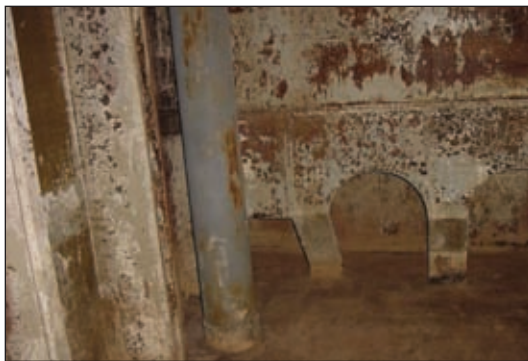
Fig. 2: The 100% solids coating can penetrate crevices formed from tightly adherent rust and old coatings. Courtesy of Van Zonderen Offshore
