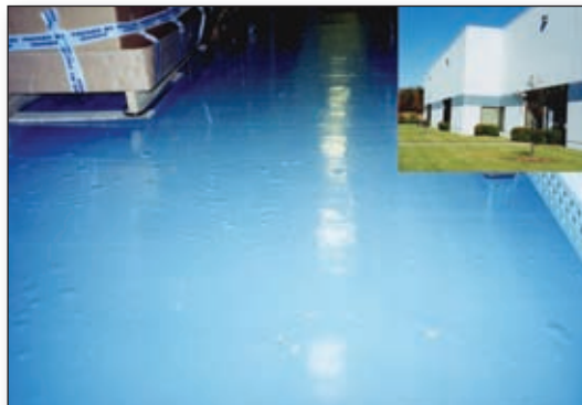
(above and below): Delamination and blistering caused by moisture in concrete. All photos courtesy of the author
