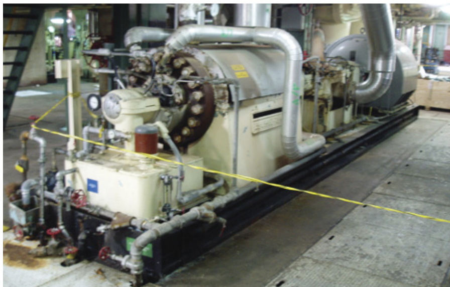
Fig. 3: Sample survey, Unit 1 boiler, feed pumps, and surrounding steel
