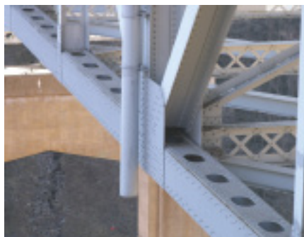
Fig. 10: Crevice connections after application of high-ratio calcium sulfonate.
