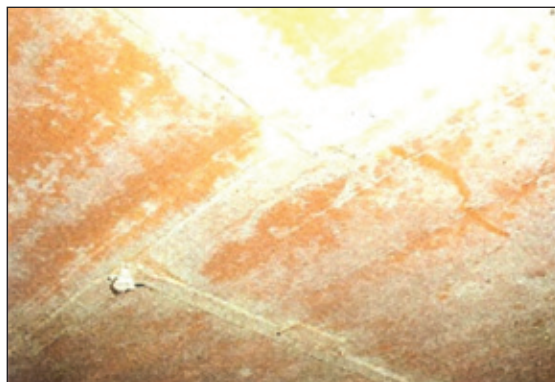
Fig. 1: Discoloration only on exposed surface of anchored PVC sheet
