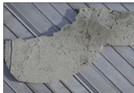
Fig. 11: Splitting of cementitious filler/surfacer applied before heated, spray-applied, 100% solids epoxy lining
