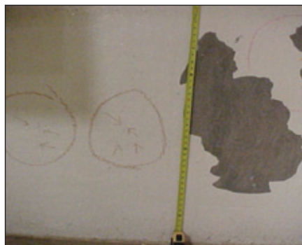
Fig. 10: Pinhole and cracking locations in heated, spray-applied 100% solids epoxy lining
