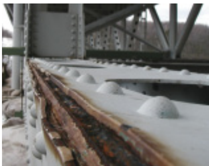
Fig. 9: Brown streaks at structure-critical connections indicate crevice corrosion.
