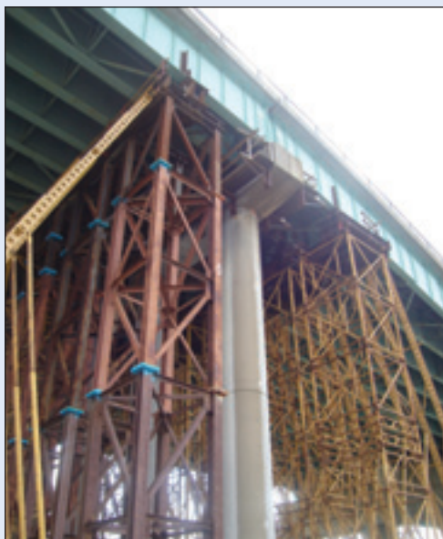
Temporary shoring during bridge repair Courtesy of PennDOT
