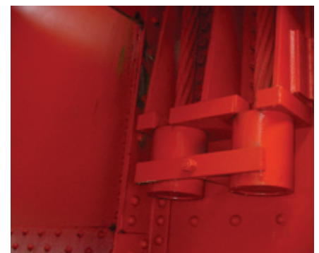
Fig. 10 (top): Suspender Socket Fig. 11 (below): Restored Socket
