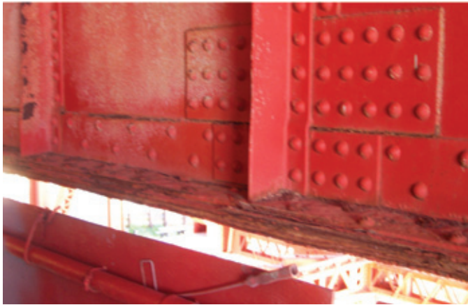
Fig. 7: Initial condition of floor beam
