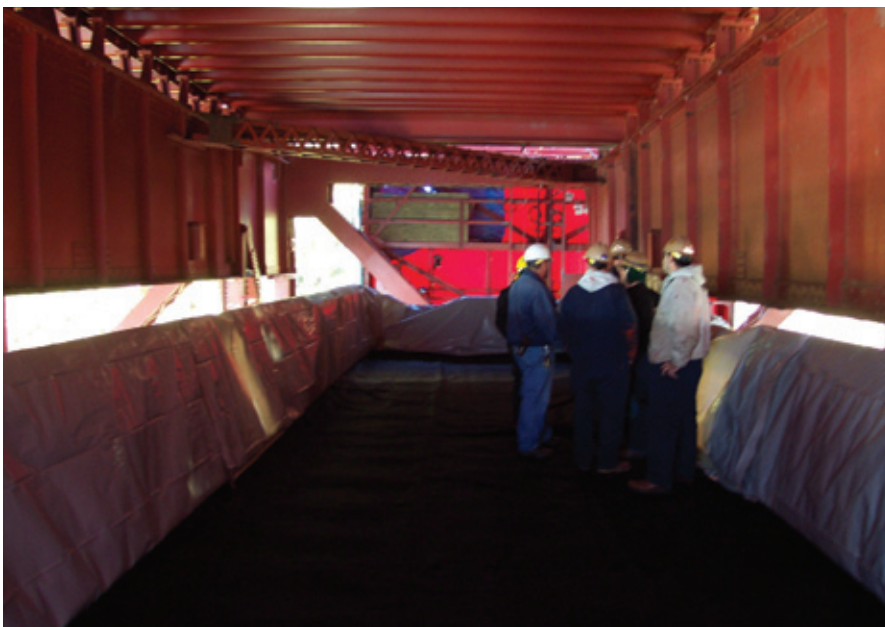
Fig. 5: UHP waterjetting containment Fig. 6 (top right): Waterjetting equipment staging
