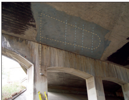
Dashed lines show the locations of wire connections on the underside of the Maryland Avenue Bridge in St. Paul, MN. Photo courtesy of Cortec Corporation
