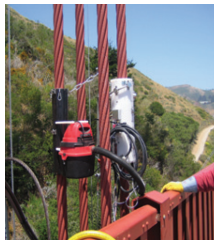
Fig. 13: Automated painting tool
