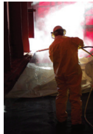
Fig. 9: Waterjetting in progress
